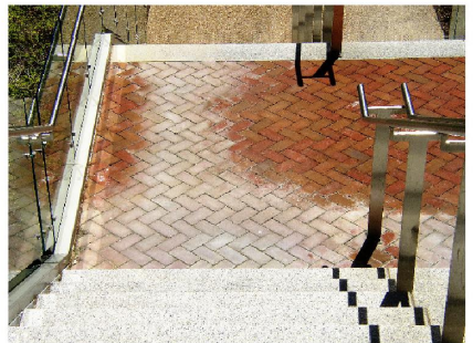
EFFLORESCENCE REMOVAL
